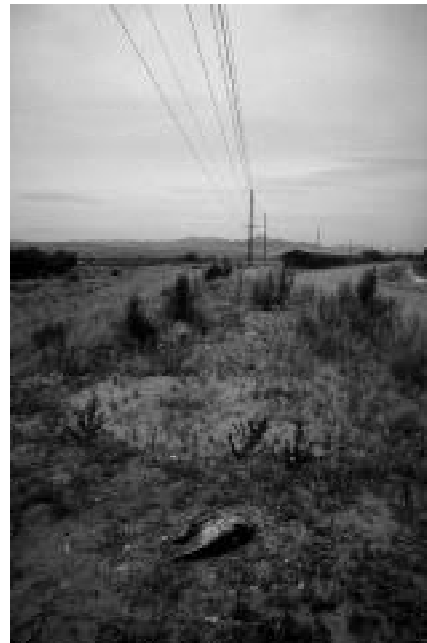
Photo 4. Electrocuted red-tailed hawk under a steel distribution underbuild mounted on a steel transmission pole.
