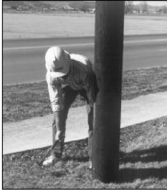
On average, most utilities inspect poles every five years.
